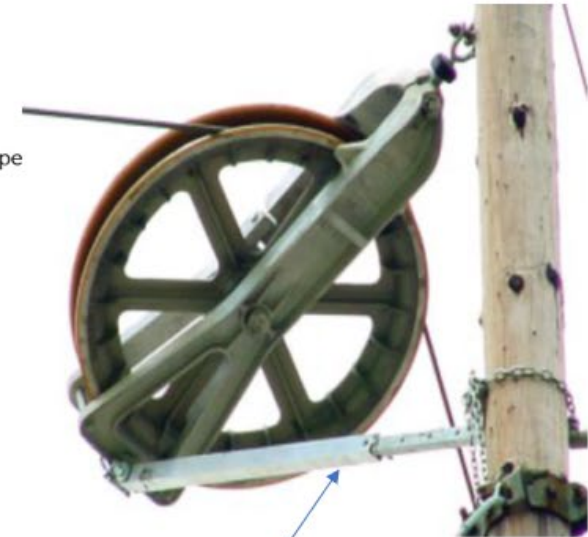
Support from underneath block
