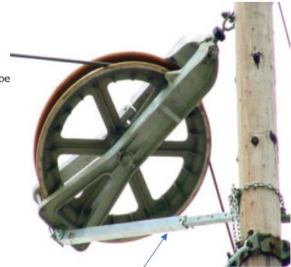
Support from underneath block
